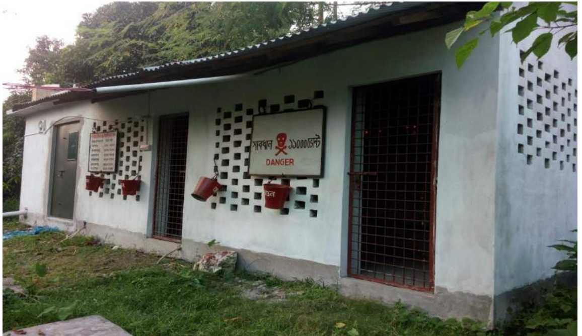
BS- own Power Sub-station for electricity supply
