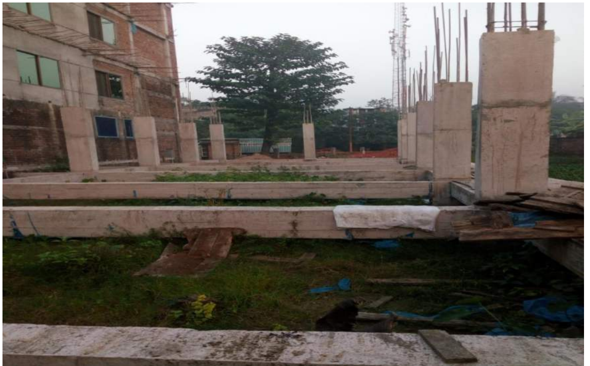
New building – under construction
